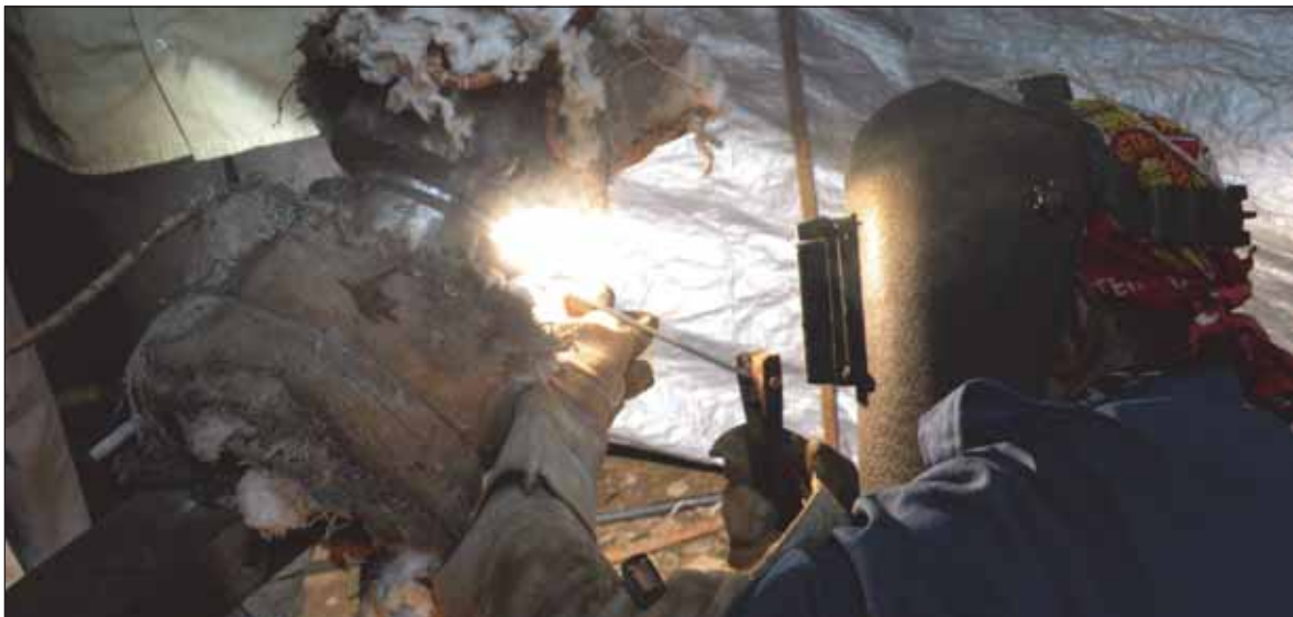
Testing of Welders at Site
